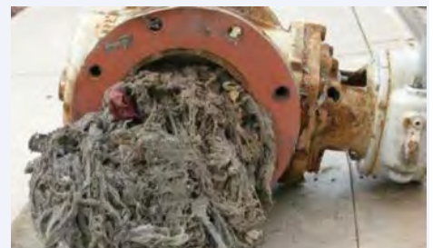
A mass of flushable and disinfectant wipes clogs a pipe.
